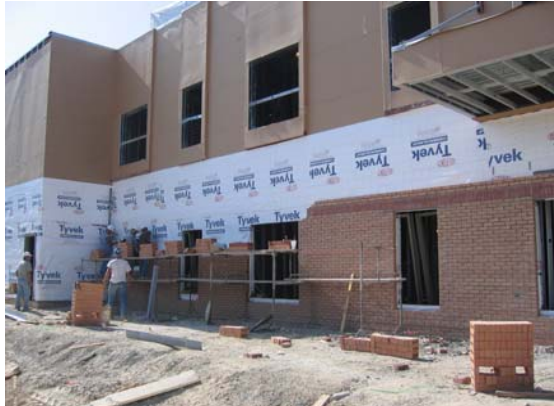
Bricklayers on the Job.
