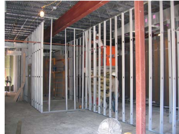
Walls taking shape
