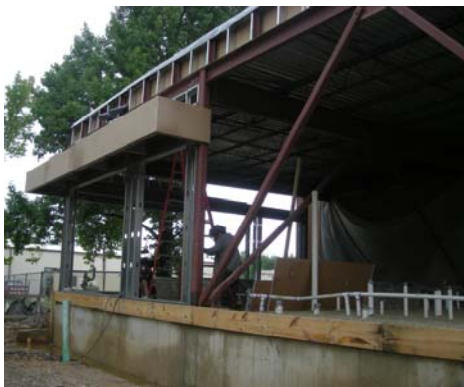
New Physical Therapy Area in Progress
