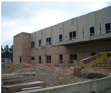
East side of new Addition taken 8/13/08
