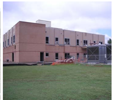
North side of new addition taken 8/13/08
