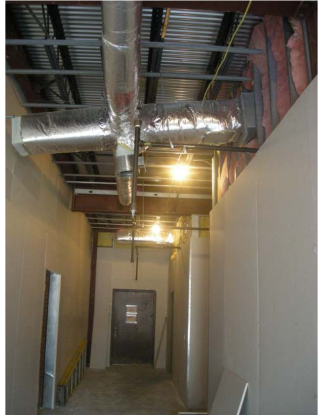
Current View of Interior hallway - North Tower
