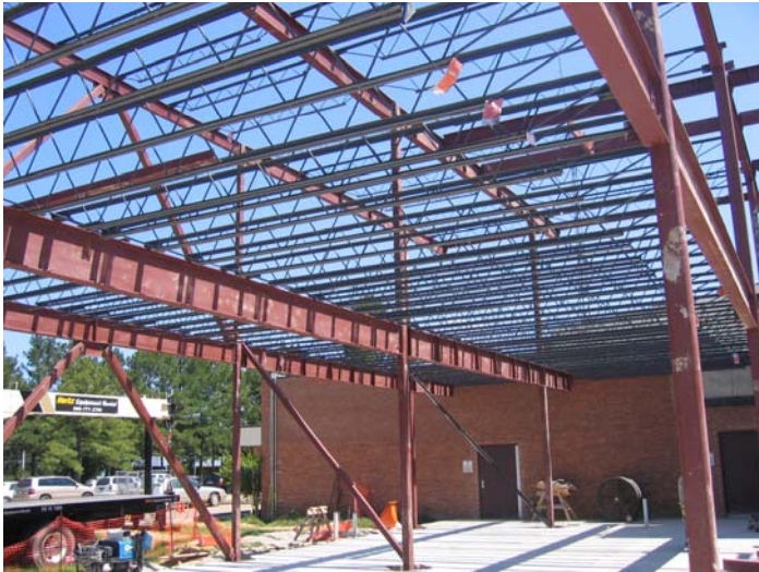
Steel going up on North Tower week of June 3rd
